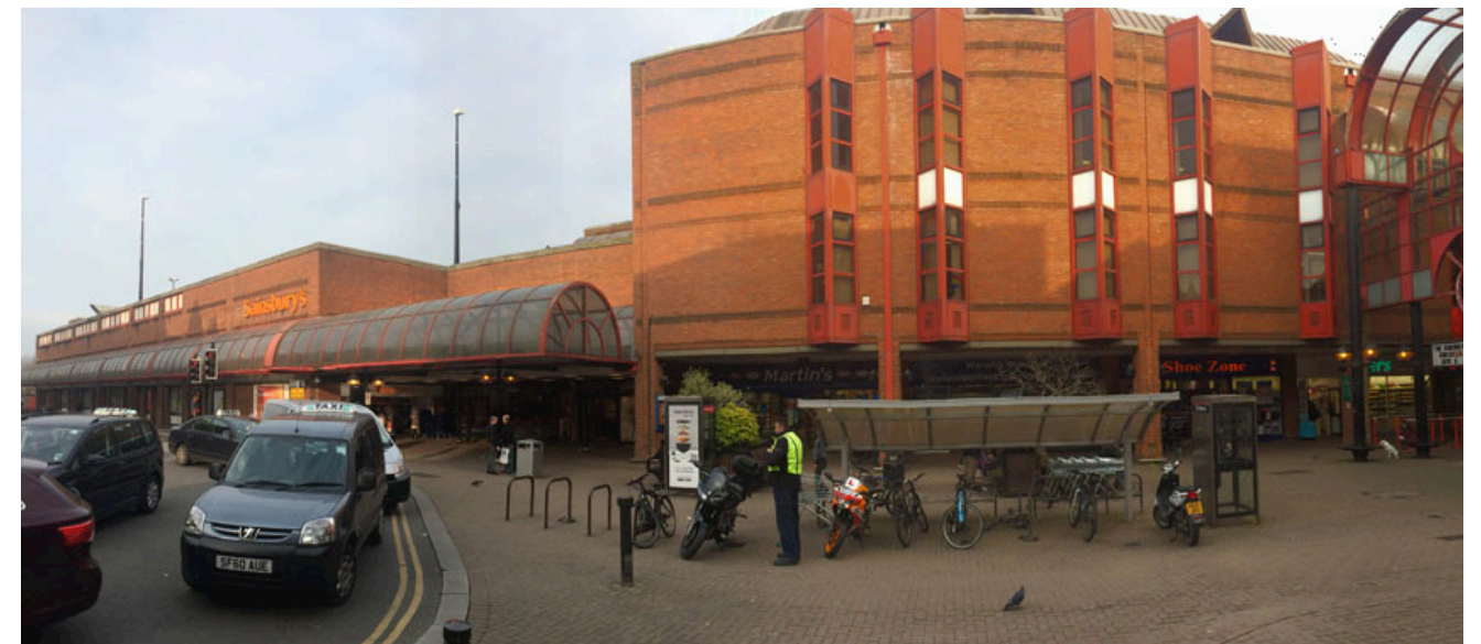
1. Existing view of London Road
